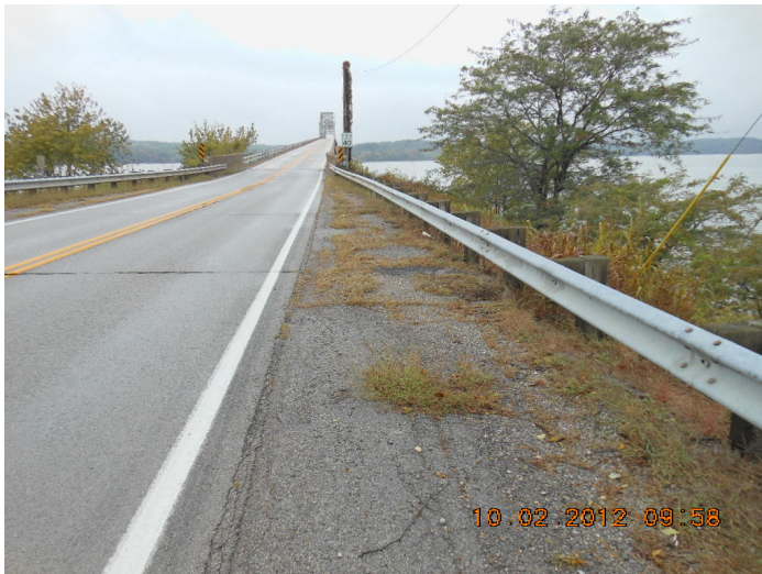
Bridge across Lake Barkley/Cumberland R. (photo courtesy Scott Cooper)
