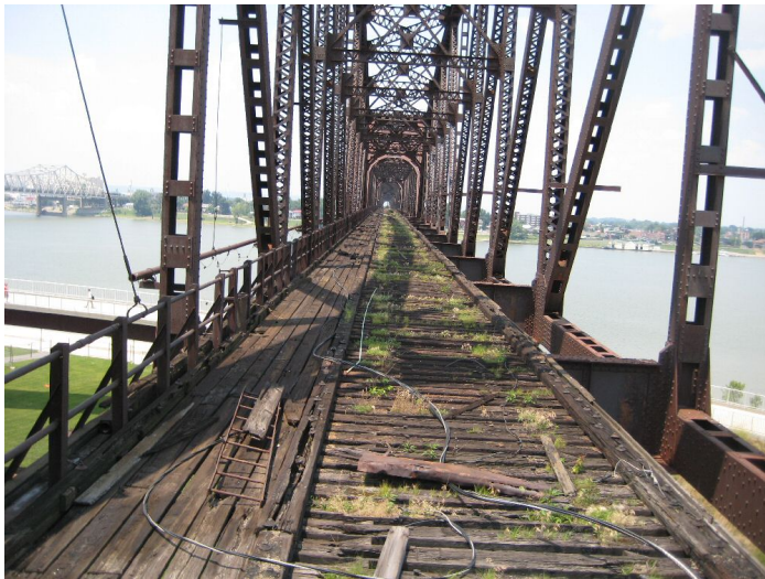
Big 4 Bridge Deck Pre-Construction (photo courtesy Andy Murphy)
