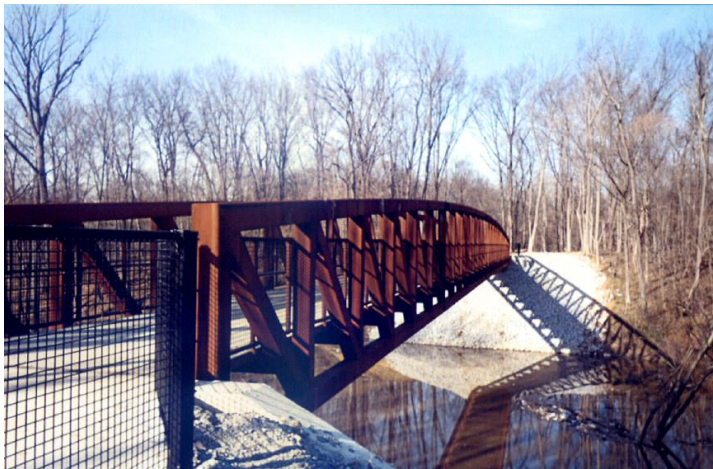
Newly-built Mill Creek Bike/Ped Bridge, Levee Trail, W Jeff. Co. (Photo courtesy Andrew Murphy)
